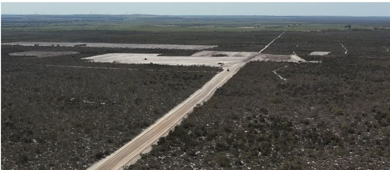
Photo 1: Atlas Mine – Access road and topsoil stripping
