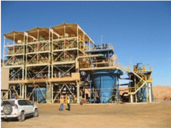
Wet Concentration Plant
