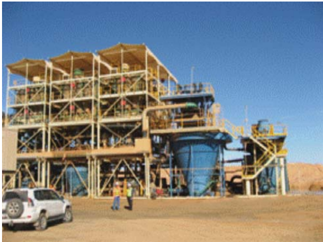
Wet Concentration Plant
