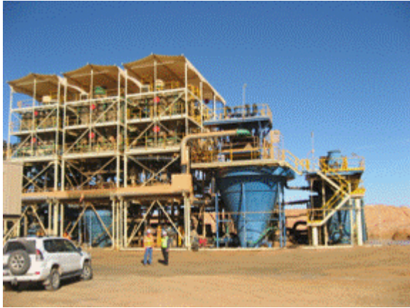
Wet Concentration Plant
