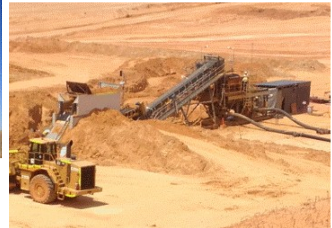
Mine Slurry Unit
